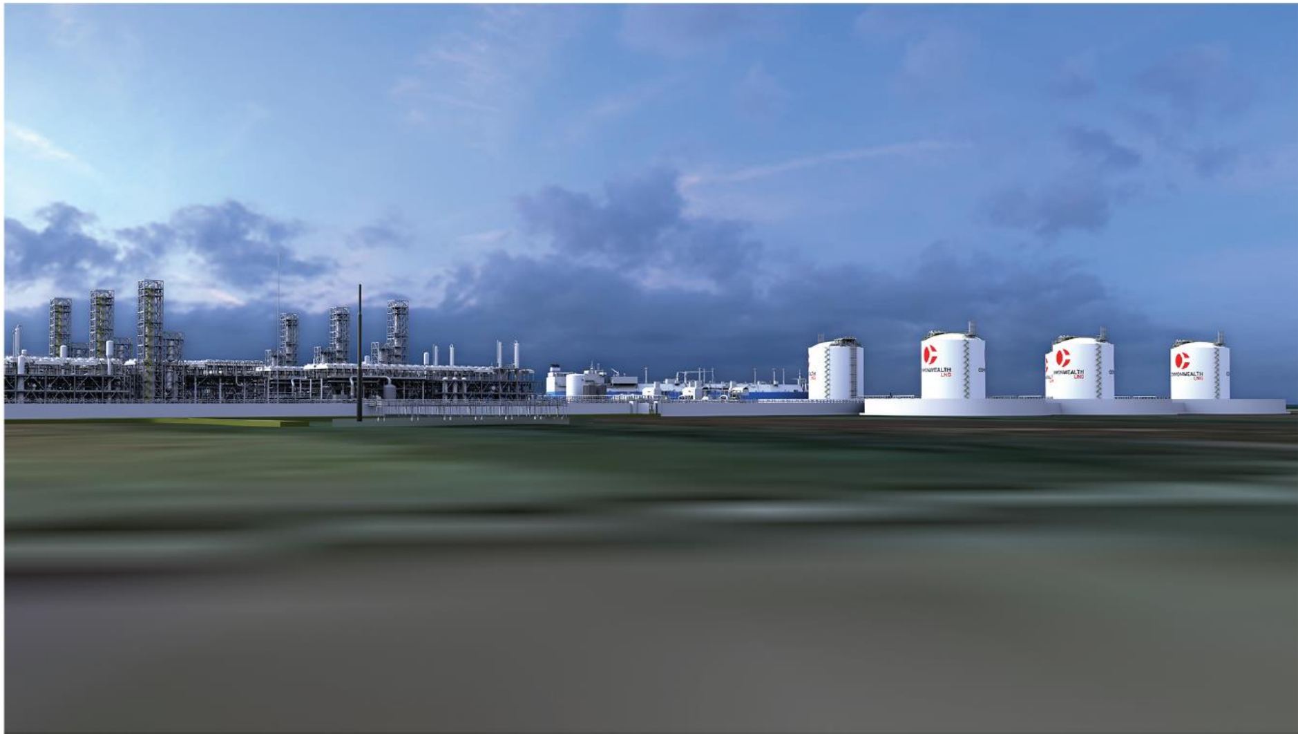
Figure E-4. Daytime rendering of the Commonwealth LNG Terminal viewed from NSA 2.
