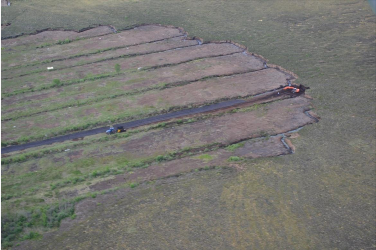
About five plots have been cut so far this year at Moneybeg bog, located on the southern shores of Lough Sheelin in Co. Westmeath/Meath. The digger and spreader were working on the day of our survey. Note the enormous spreading area below, comprising turf from several plots.
